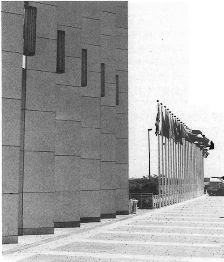
The base of the soaring Amoco Building. North Carolina granite has replaced the shimmering Carrara marble that proved inadequate in this blustery, exposed site.
