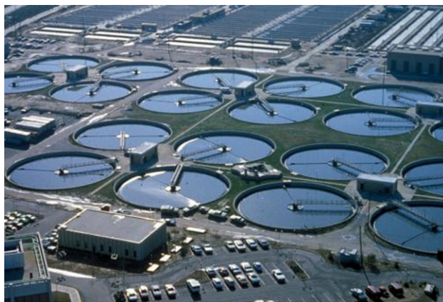
Figure 15.6 Wastewater treatment facilities, such as this one, remove contaminants from wastewater before the water is released back into the natural environment. (credit: "eutrophication&hypoxia"/Wikimedia Commons)
