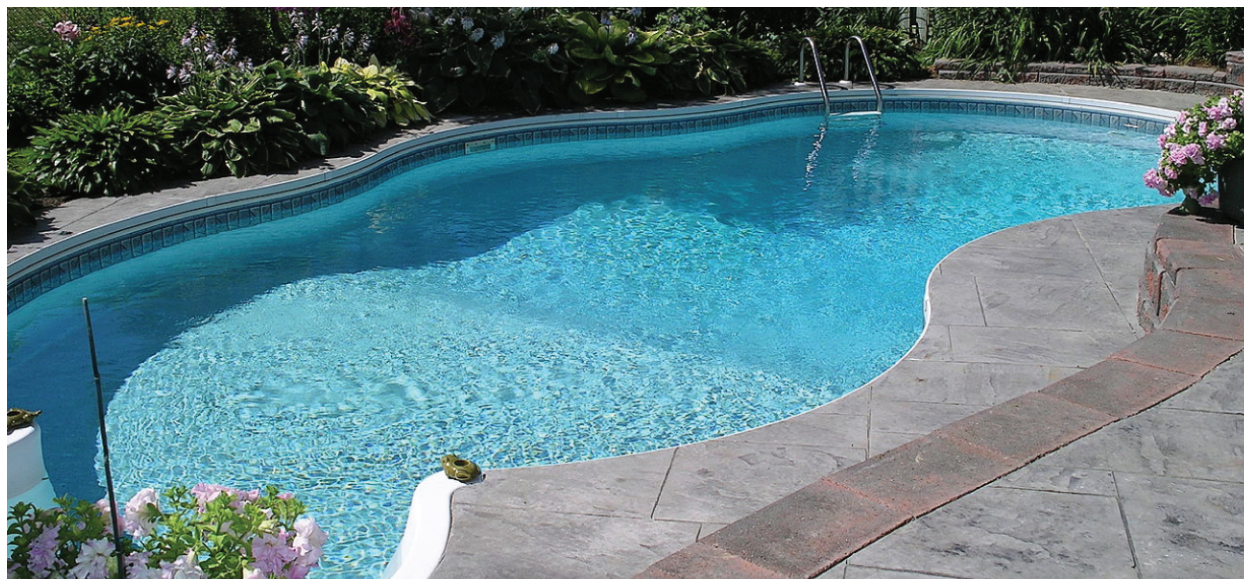
Figure 6.1 The water in a swimming pool is a complex mixture of substances whose relative amounts must be carefully maintained to ensure the health and comfort of people using the pool. (credit: modification of work by Vic Brincat)
