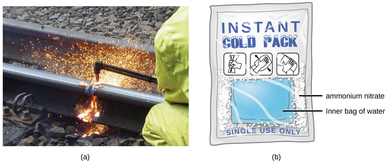
Figure 9.7 (a) An oxyacetylene torch produces heat by the combustion of acetylene in oxygen. The energy released by this exothermic reaction heats and then melts the metal being cut. The sparks are tiny bits of the molten metal flying away. (b) A cold pack uses an endothermic process to create the sensation of cold. (credit a: modification of work by “Skatebiker”/Wikimedia commons)
