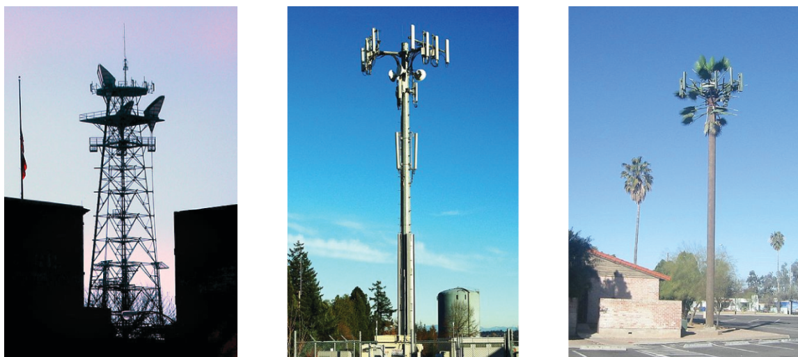
Figure 3.4 Radio and cell towers are typically used to transmit long-wavelength electromagnetic radiation. Increasingly, cell towers are designed to blend in with the landscape, as with the Tucson, Arizona, cell tower (right) disguised as a palm tree. (credit left: modification of work by Sir Mildred Pierce; credit middle: modification of work by M.O. Stevens)
